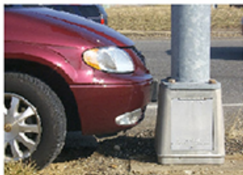
Notice height of car bumper before impact. Impact is absorbed by cast aluminum base, not pole.
